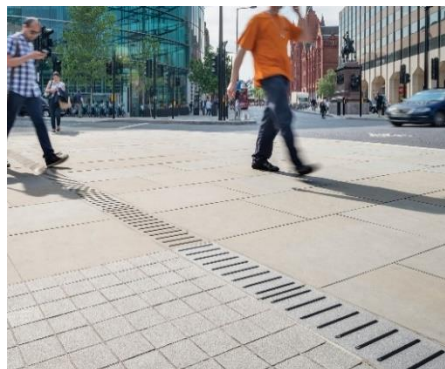
Photograph 45 - Example of a Channel Drain
