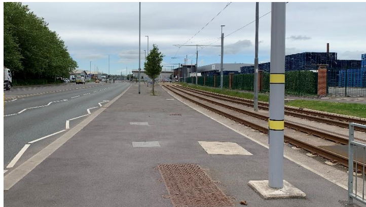
Photograph 18 - Existing Village Way
