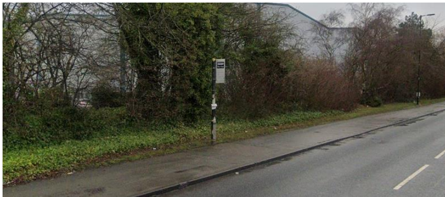
Photograph 32 - Existing Bus Stop, Ashburton Road West
