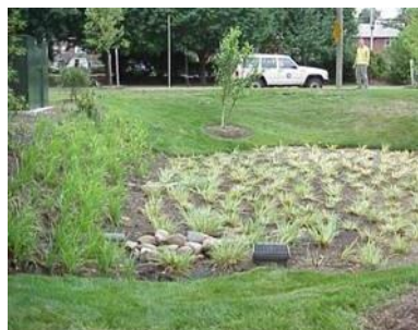
Photograph 38 - Example Bio-Retention Area
