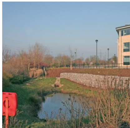
Photograph 42 - Example of Detention Basin
