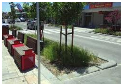
Photograph 39 - Example Bio-Retention Tree Pit
