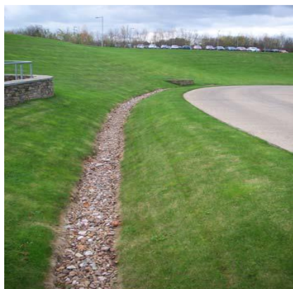
Photograph 41 - Example of an Infiltration Trench
