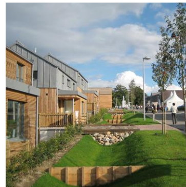
Photograph 40 - Example of a Swale
